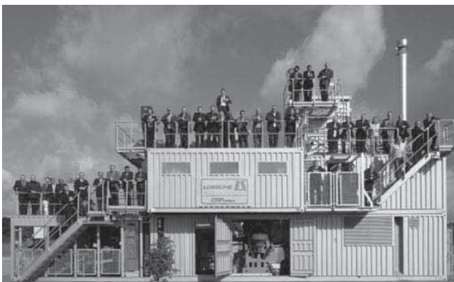
The mobile grinding plant in Jasien, Poland.
